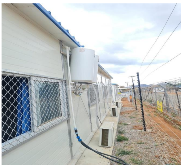
Cabins with geysers and air conditioning. To the right is the electric fence
