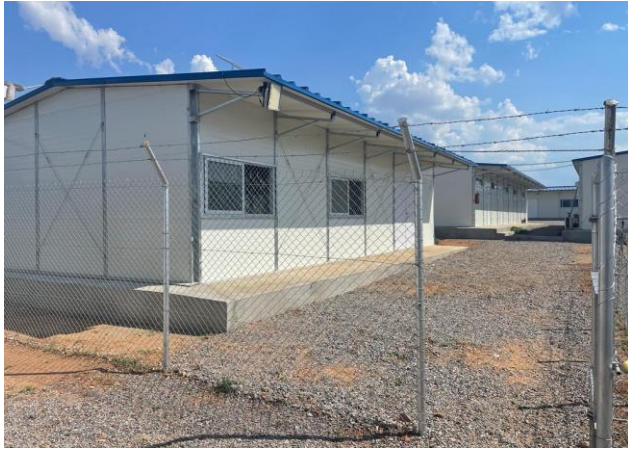
Entrance of the accommodation camp from Contractor's site office
