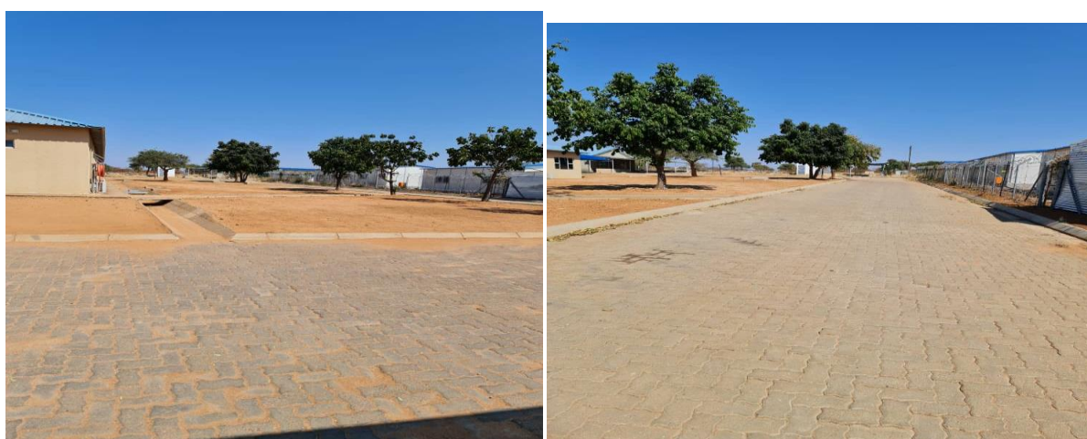
View of Supervising Engineers' building to the left and Contractor's camp site to the right
